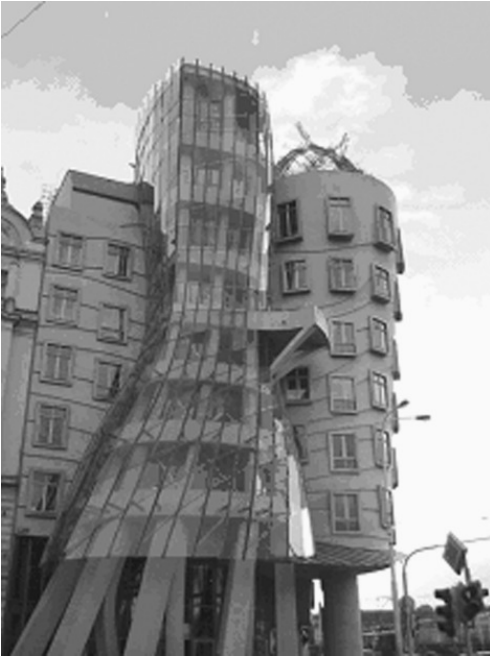
Frank Gehry's "Ginger and Fred" Building in Prague. Photo by Garrett Weinberg.
